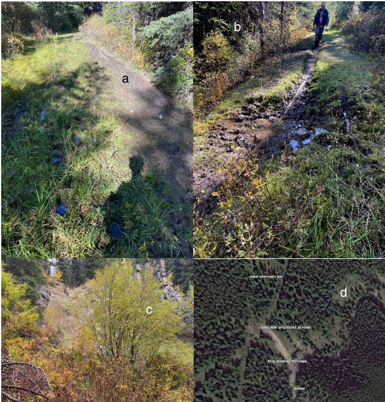
Figure A4. Groundwater and surface flow are intercepted by the legacy roadbed, turning it into an active watercourse (a, b). The water has been directed to a spot, which became saturated and failed, causing a landslide that sent debris into Loomis Creek channel, and upstream in the creek (c, d). Photos (a, b) M. Coombs, (c) D. Mayhood, (d) Google Earth imagery 2013.08.31
