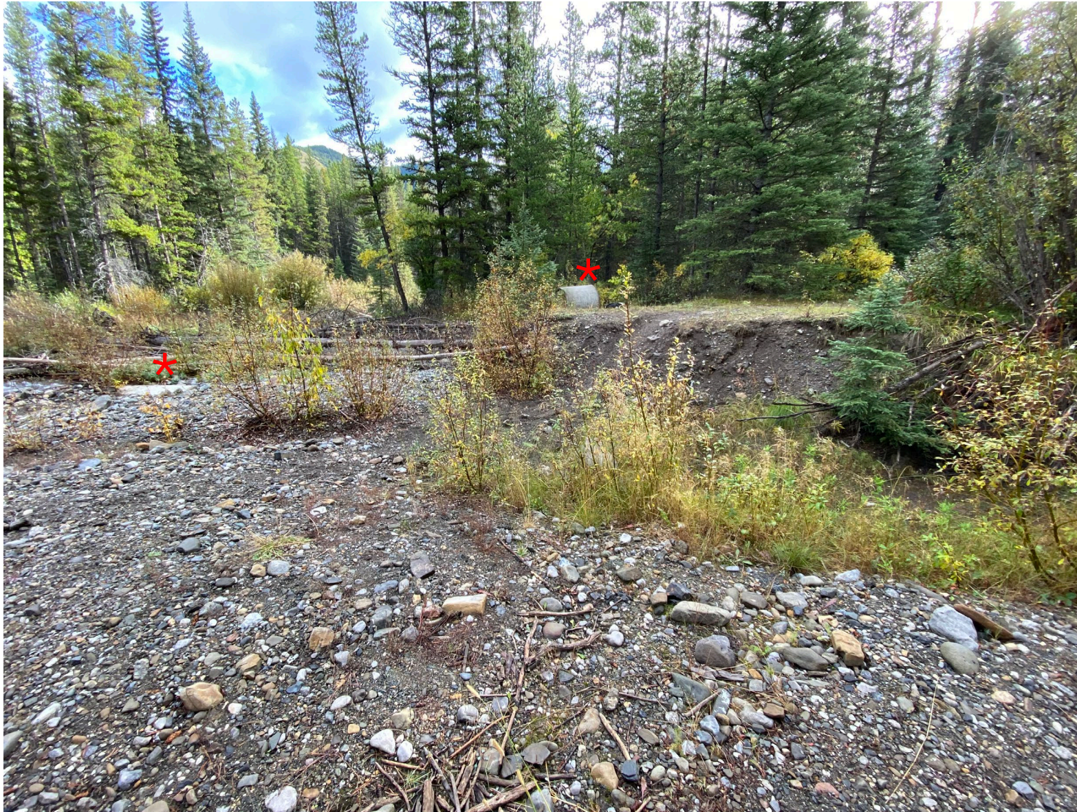
Photo 1. Loomis Creek Blowout Crossing showing channel avulsion and pieces of a concrete culvert (*).
