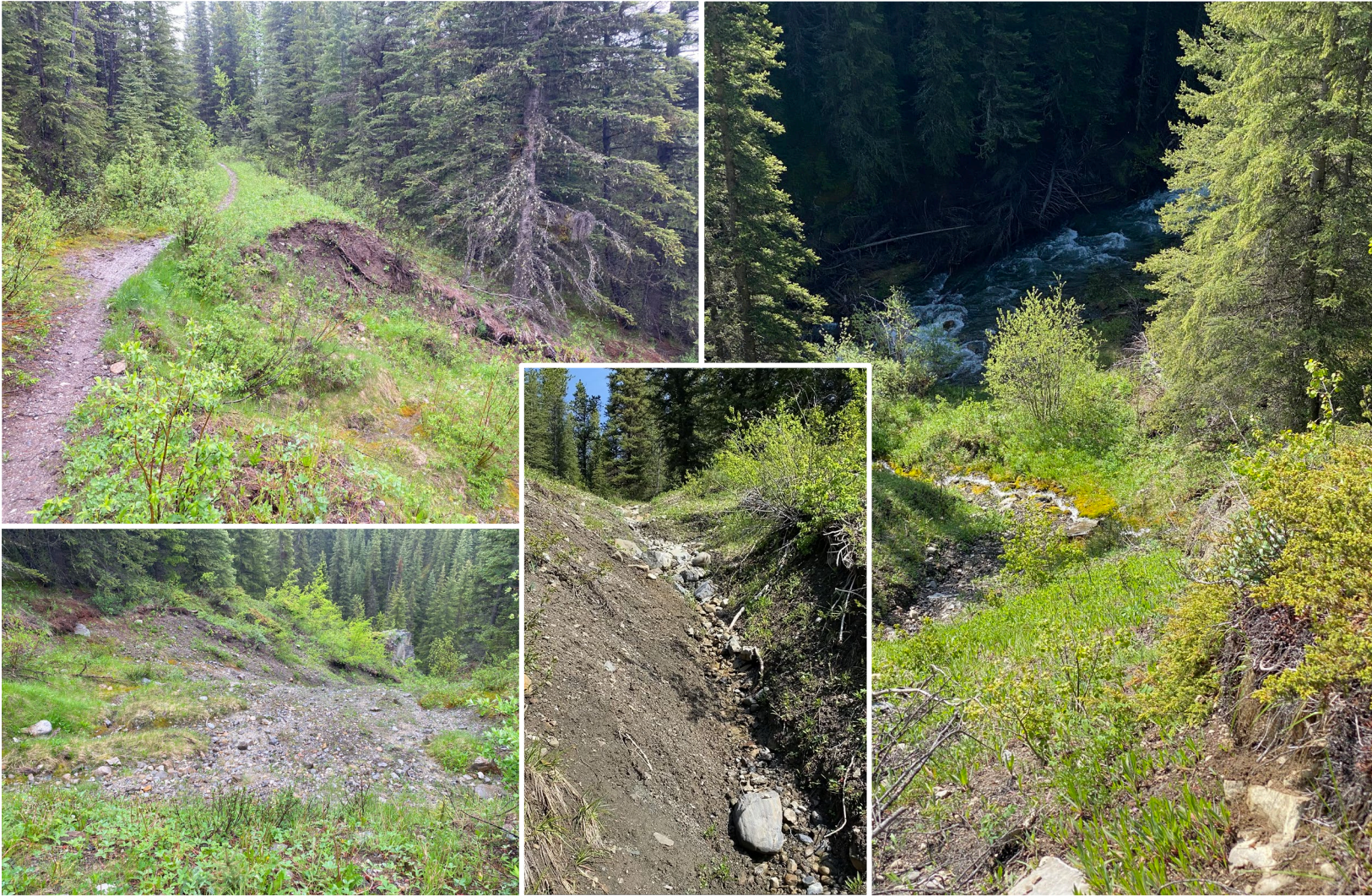
Photo 21. Section of historical logging road situated on saturated soils that slid into Loomis Creek.
